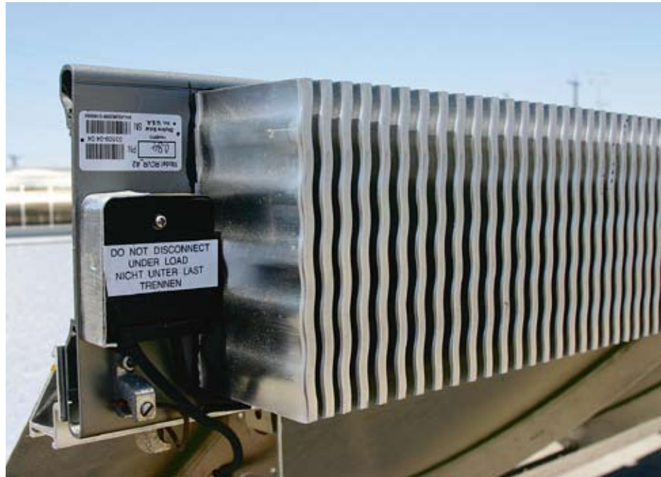
The purpose of the cooling fins at the back is to improve the temperature behaviour of the monocrystalline cells.
